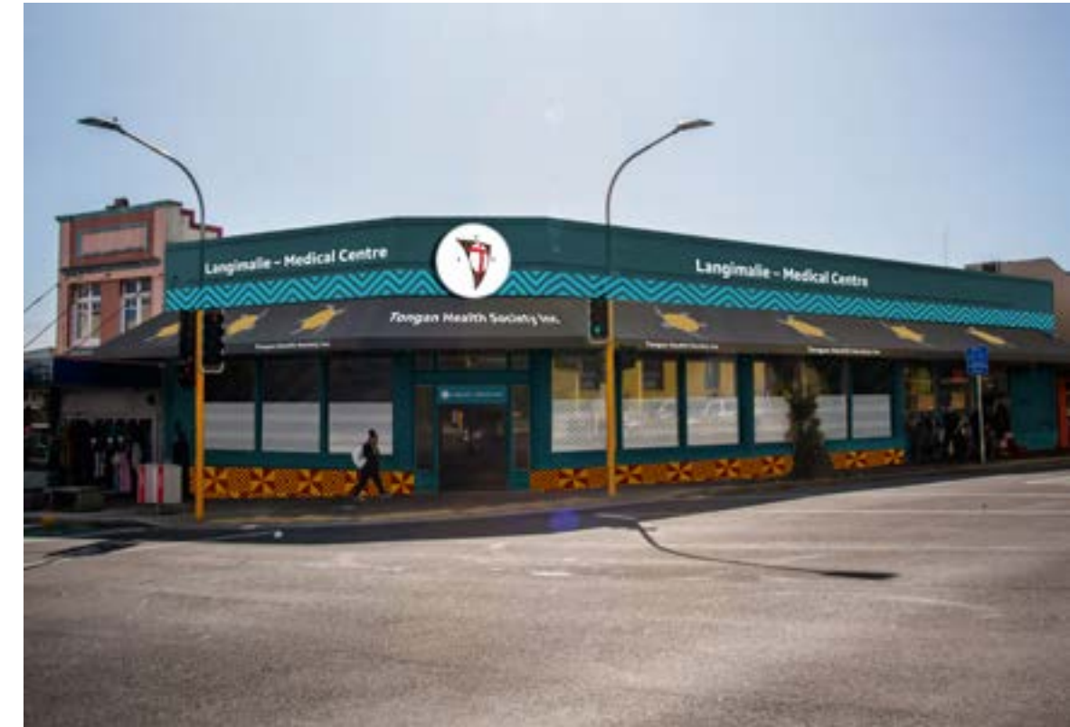
▲ Location of Langimalie medical centre in Ōtāhuhu.
